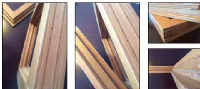
Two 5mm Cork layers in a window frame of 500 x 500mm
